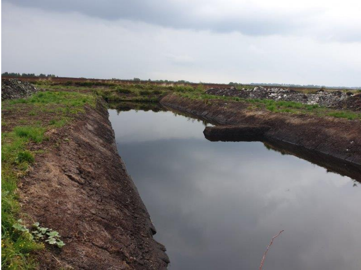
Sedimentation pond at peat extraction site. Photo: Florence-Renou Wilson
